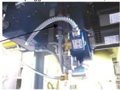
✓ Inspect the pipe that the cad cell attaches to, and if dirty or dusty, clean with a rag to remove buildup.
