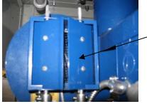
Inspect-air doors and fan for buildup of dust. Note air door setting, blow out any buildup, and set air door to original setting. If in doubt as to correct settings, contact a local distributor to perform a flue gas analysis, or consult Sioux Corp. for assistance.
